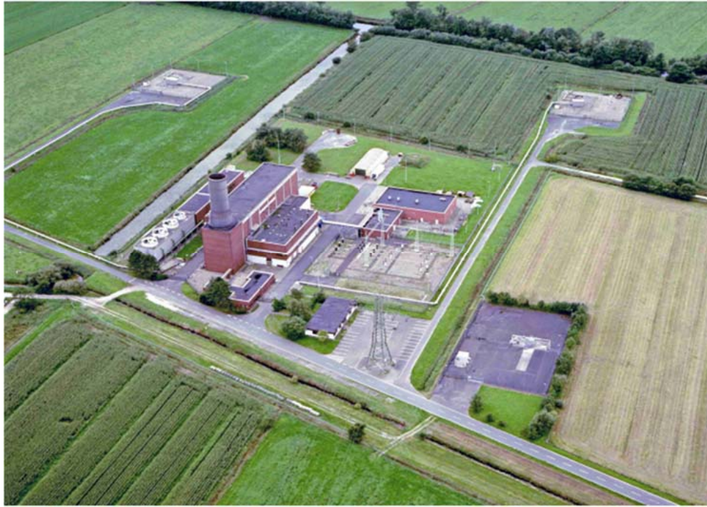
Fig. 7. The Huntorf CAES Plant (Source: DOE Global Energy Storage Database).
