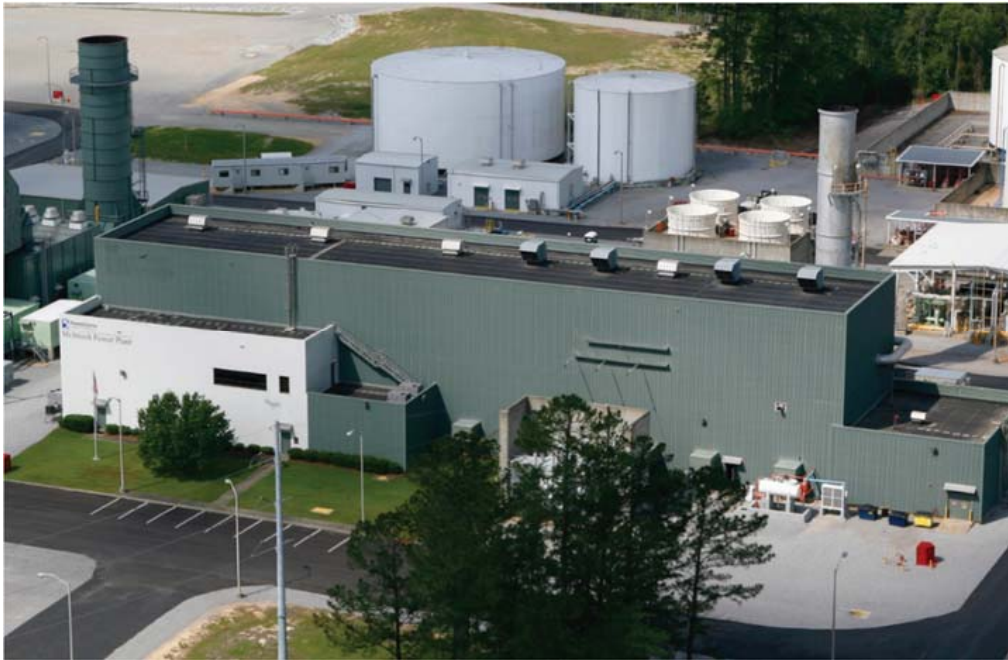
Fig. 8. The McIntosh CAES Plant (Source: DOE Global Energy Storage Database).
